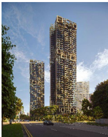
17_DAM_IHP26-27_MVRDV_Irwell-Hill-Residences_Foto- Finbarr Fallon. Image courtesy of MVRDV_Foto-Finbarr Fallon. Image courtesy of MVRDV
