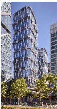
26_DAM_IHP26-27_Skidmore-Owings-&-Merrill_Sany-IROOTECH-Headquarters_Foto-Dave-Burk_Copyright-SOM Skidmore, Owings & Merrill, Chicago IL, USA
