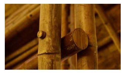
Connection details of bamboo joinery
