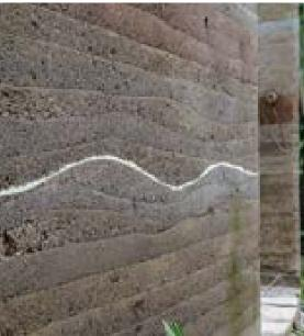
Close-up view of the wall using rammed earth construction, showing the striated and polychromatic layers of compacted earth.
