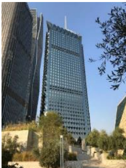
09_Dominique Perrault Architecture_European Court of Justice_Luxembourg_Michel Denancé Foster + Partners, London, Großbritannien: Samba Bank HQ Tower, Riad, Saudi Arabien Foto: Foster + Partners
