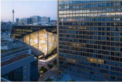
OFFICE FOR METROPOLITAN ARCHITECTURE (OMA) Axel-Springer-Neubau, Berlin Foto: Laurian Ghinitoiu
